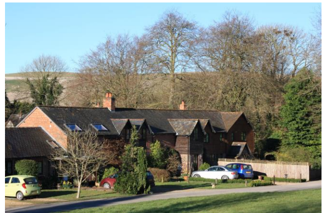
Sympathetic conversion of farm buildings at former Manor Farm, Brixton Deverill
